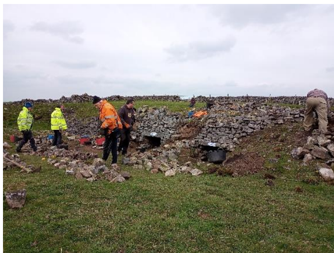
Photograph of limekiln restoration at Alsop Moor
